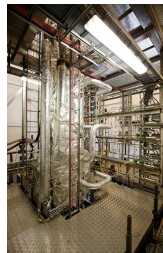
Fig. 5. Mid-section of the 150 kW CLC reactor system at SINTEF Energy Research.
